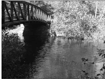
A graceful footbridge matches the terrain at Killens Pond.
